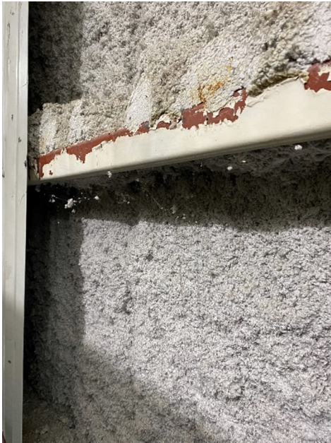
Figure 2-17 Cellulose Applied Insulation
