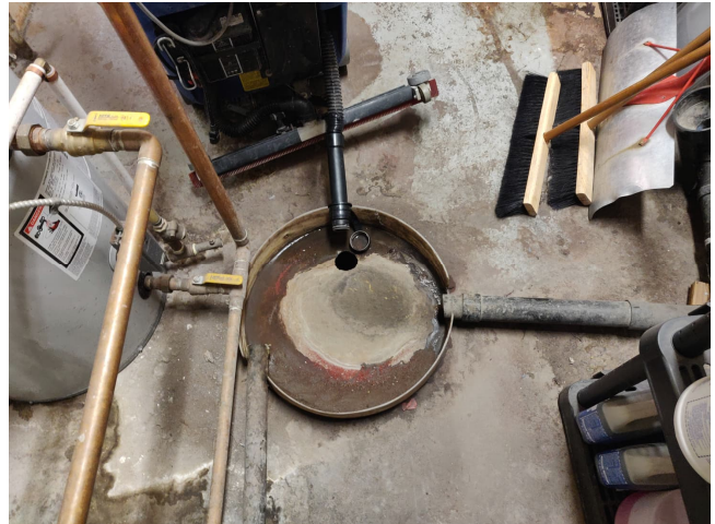
Figure 4-23 South Mechanical Room Floor Drain
