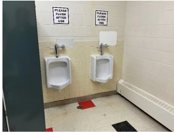
Figure 2-43 Vinyl Tile in Washroom
