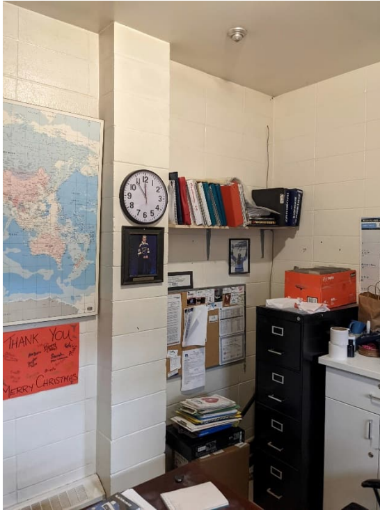
Figure 3-4 400 mm x 400 mm Masonry Pilaster in South wall
