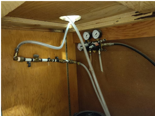
Figure 4-18 PEX Tubing Serving Coffee Equipment in Concession Area
