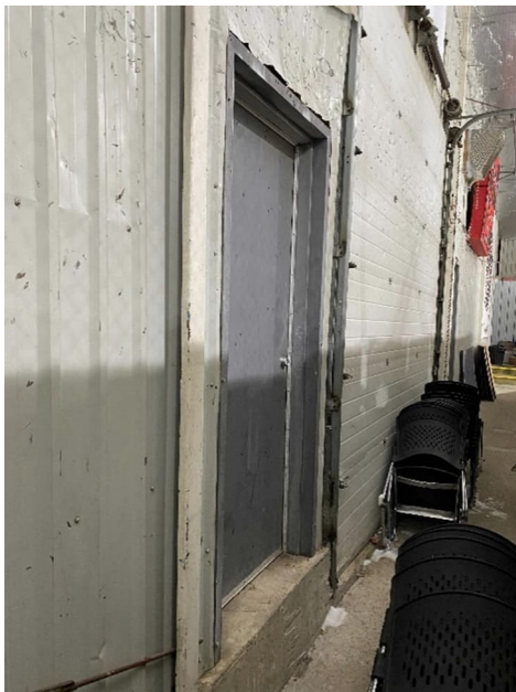
Figure 2-34 Exit Door Elevated off Ground
