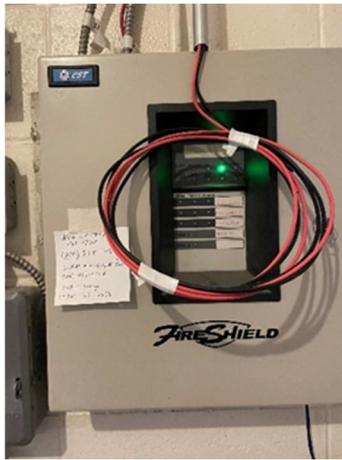
Figure 5-14 New Equipment is Tamper Resistant
