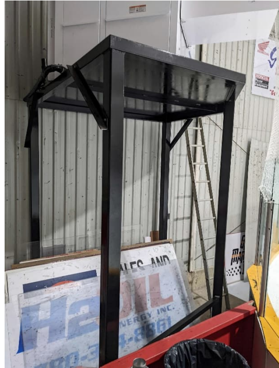
Figure 3-45 Northwest Dehumidifier Steel Frame
