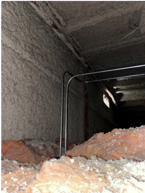
Figure 2-13 Cellulose Insulation Visible on Fiberglass Insulation
