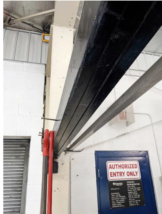
Figure 3-49 Arena Wood Beam Retrofit
