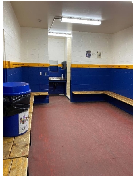
Figure 2-40 Typical Dressing Room Flooring
