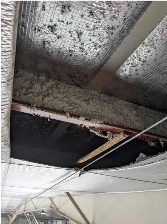
Figure 3-35 Rod and Turnbuckle Pre-Engineered Brace, Minor Corrosion
