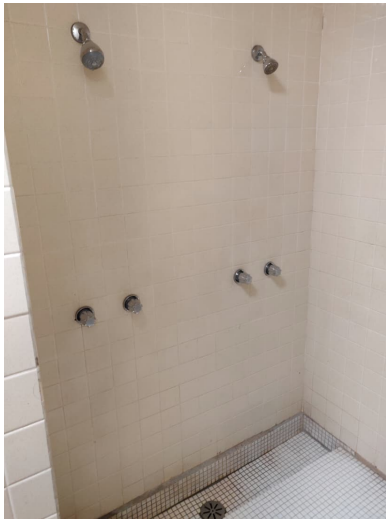
Figure 4-10 Typical Shower in Original Building Area
