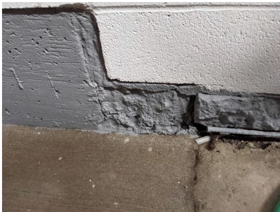
Figure 3-16 Irregular/Poor Transition in Zamboni Room Wall
