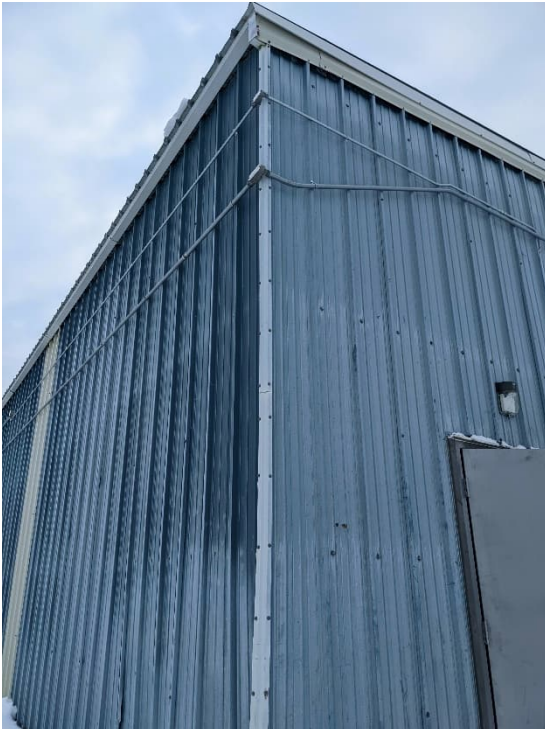
Figure 3-37 Corrugated Siding at Northeast Corner
