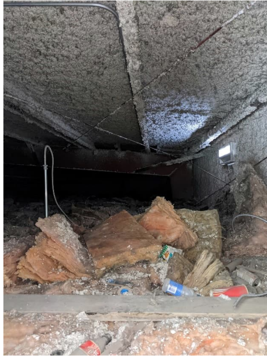
Figure 3-3 Garbage in Space Between High-Ceiling and Pre-Engineered Roof Above
