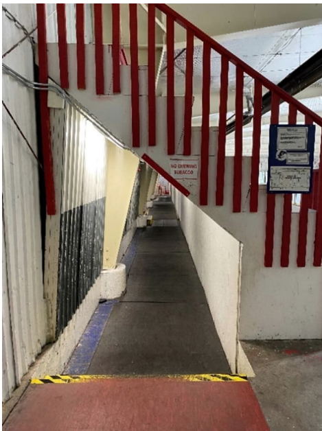
Figure 2-26 Underside of Bleacher
