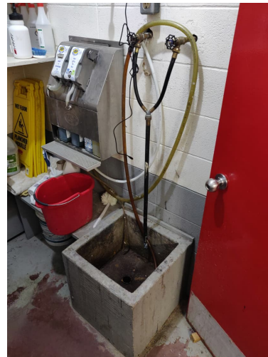
Figure 4-19 Mop Sink in Original Building Area
