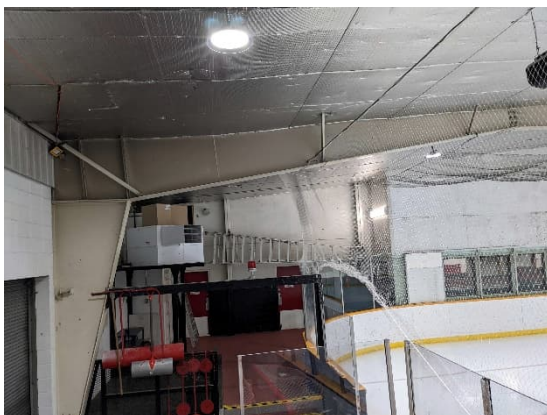
Figure 3-31 Steel Pre-Engineered Framing
