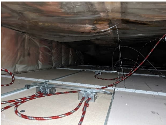
Figure 3-1 Wood-Framed Space Between High-Ceiling and Dropped Ceiling
