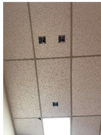
Figure 5-15 New Isolation Modules
