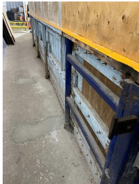
Figure 2-22 Patches in Concrete
