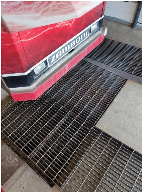
Figure 4-22 Zamboni Room Trench Drain
