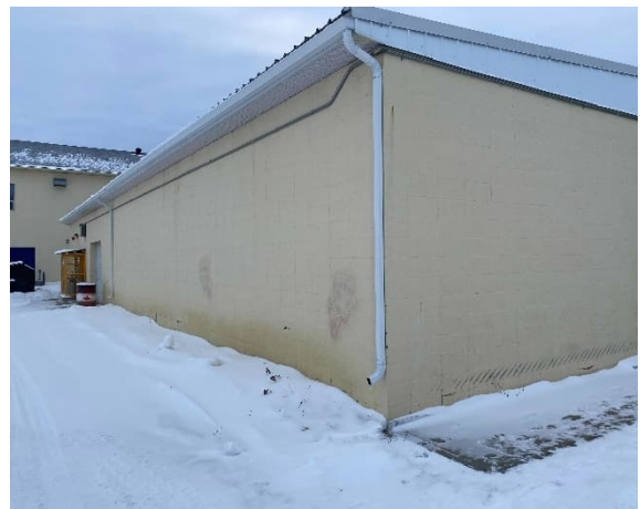
Figure 2-18 Exterior of the New Addition
