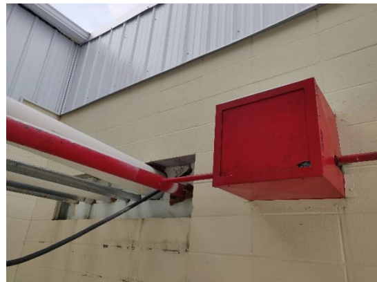
Figure 3-13 1,600 mm x 400 mm Opening Near Condensing Unit
