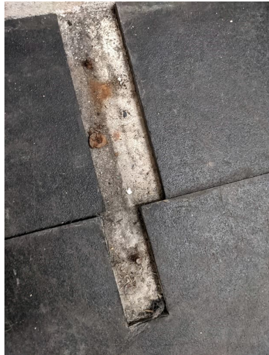
Figure 3-21 Abandoned Base Anchorage in Dressing Room 5
