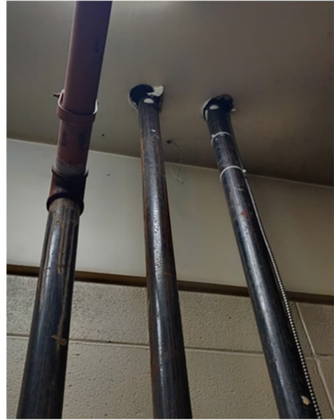
Figure 4-52 Gap in Fire Separation at Piping Through Ice Plant Machine Room Wall (Typical)
