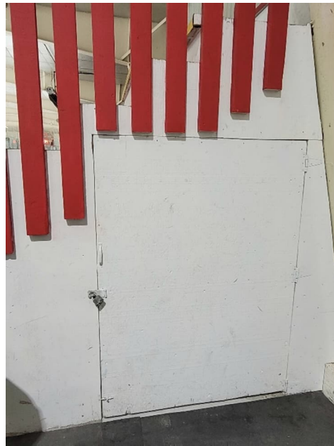
Figure 2-29 Access Gate to Storage Under Bleachers
