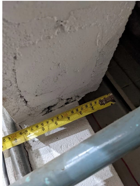
Figure 3-19 70 mm Masonry Wall Offset
