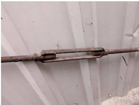
Figure 3-35 Rod and Turnbuckle Pre-Engineered Brace, Minor Corrosion
