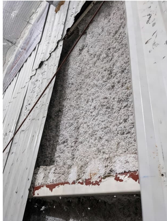
Figure 3-38 Steel Girt at Interior Exposed Panel
