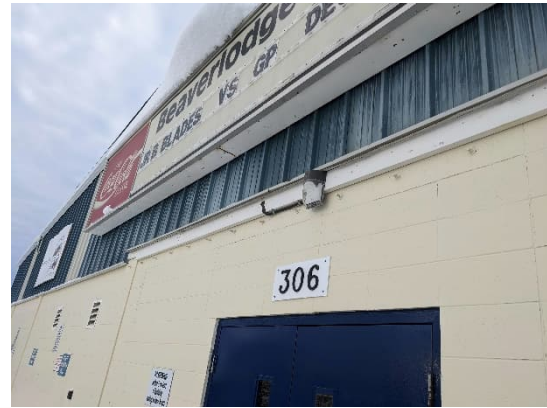
Figure 3-5 Steel Through-Bolts Above Main Entrance
