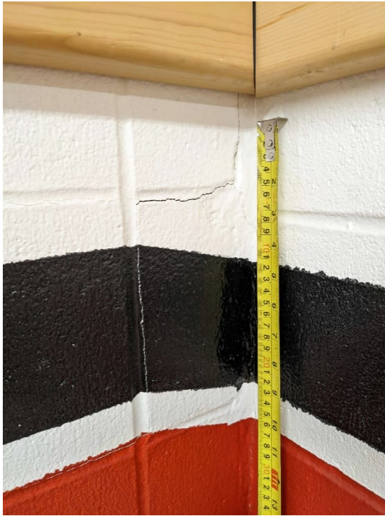
Figure 3-16 Irregular/Poor Transition in Zamboni Room Wall
