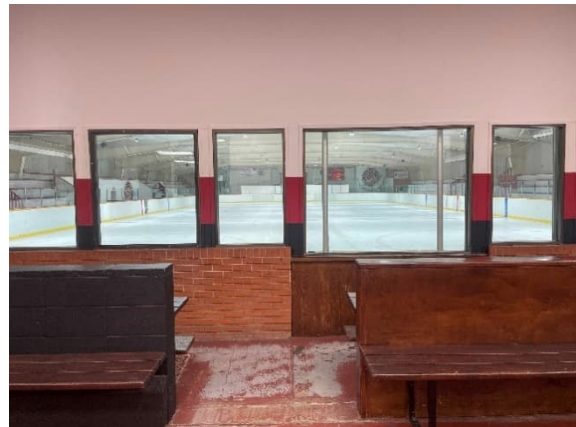
Figure 2-42 Damaged Epoxy Flooring
