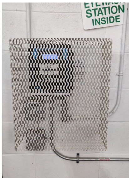
Figure 4-43 Gas Detection System and Eyewash Sign Outside Machine Room
