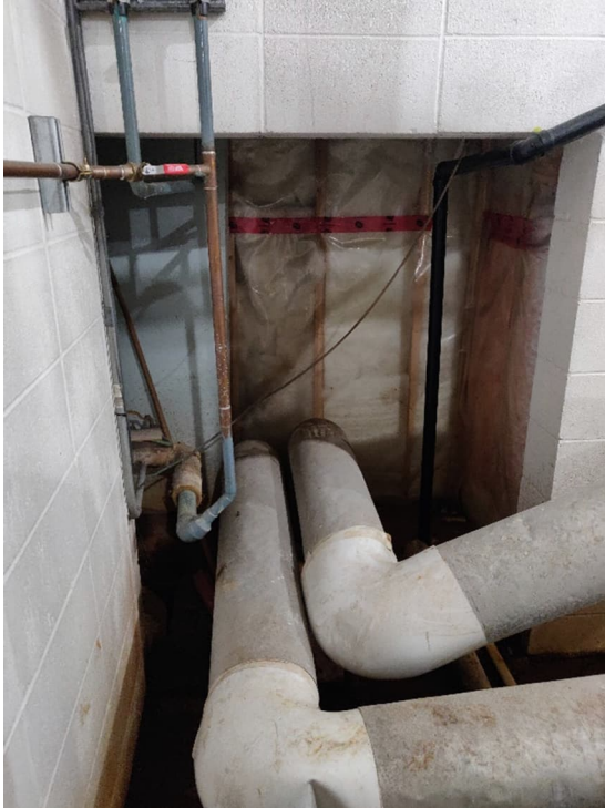
Figure 3-18 Masonry Opening in Southwest Corner of Ice Plant
