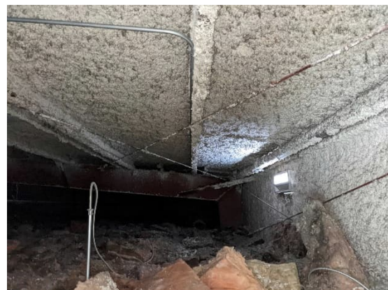
Figure 3-32 Pre-Engineered Steel Framing Above Lobby
