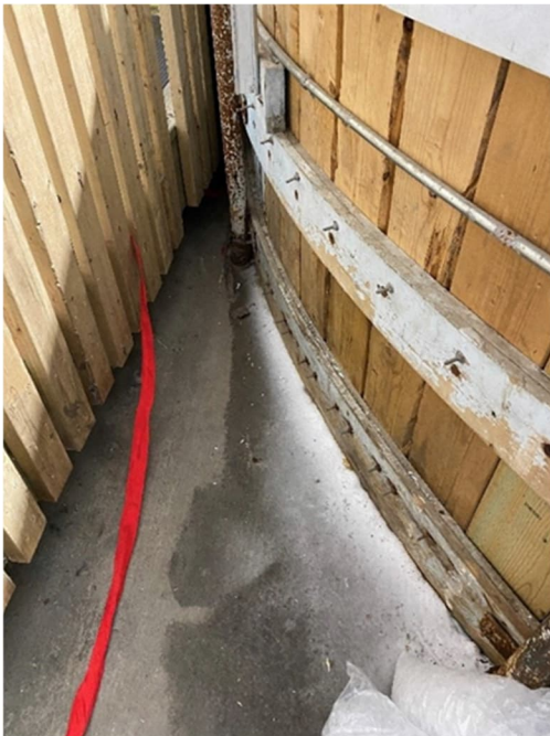
Figure 2-23 Ice Build-Up Outside of Dasher Boards
