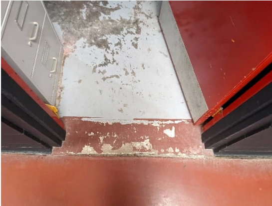
Figure 3-8 Typical Doorway Threshold at Interior Masonry Wall
