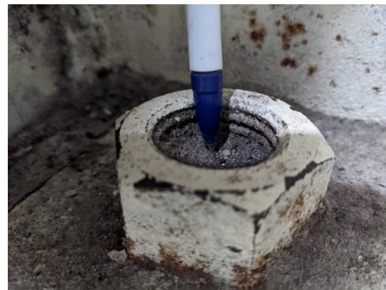
Figure 3-41 400 mm Tall Curb and Slab Interface Debonding
