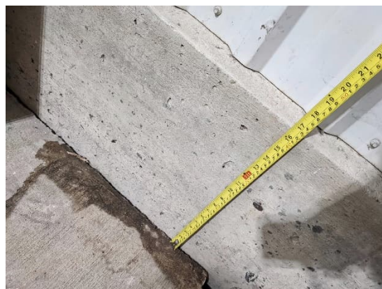
Figure 3-41 400 mm Tall Curb and Slab Interface Debonding
