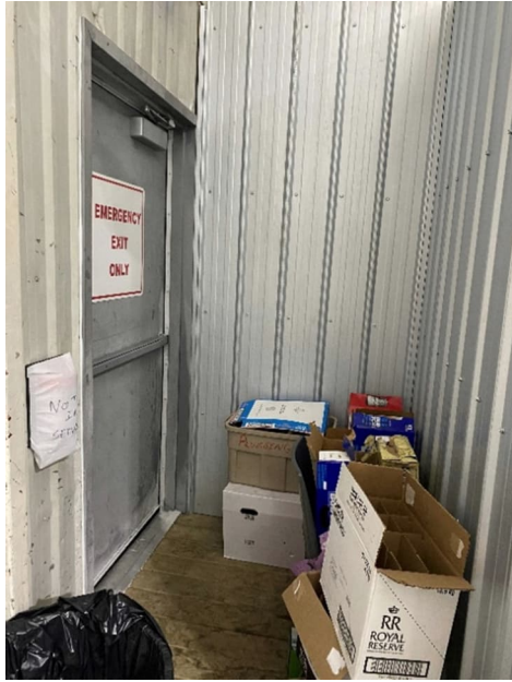
Figure 2-34 Exit Door Elevated off Ground
