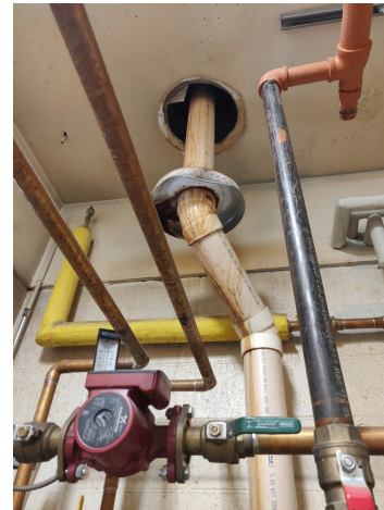
Figure 4-35 Typical Circulator Pump in South Mechanical Room
