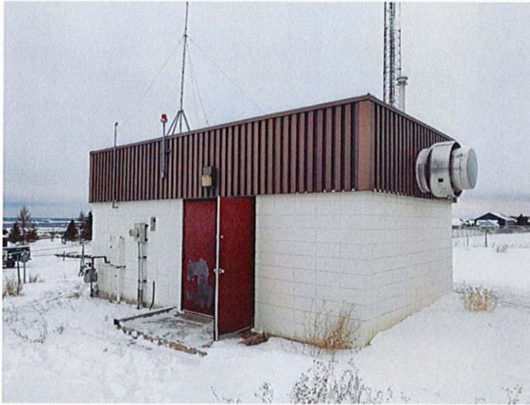
Figure 3-1 Farm/Old Town Pumphouse
